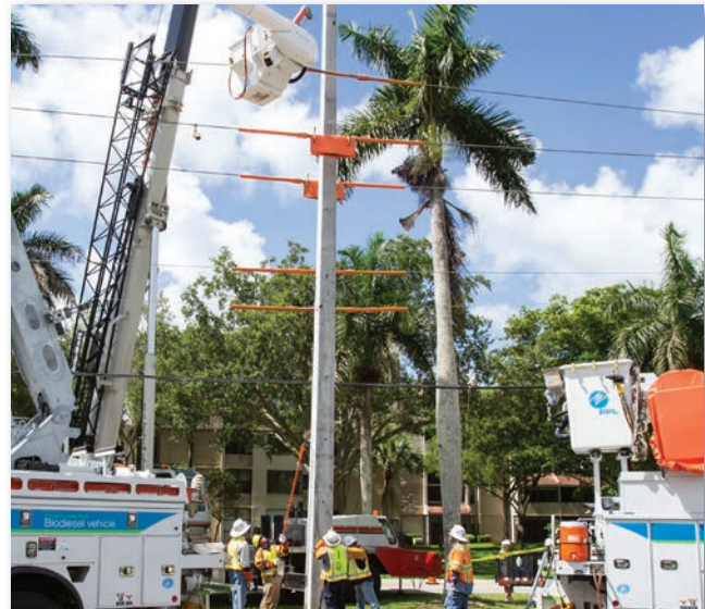
Wooden poles are replaced with concrete poles.
