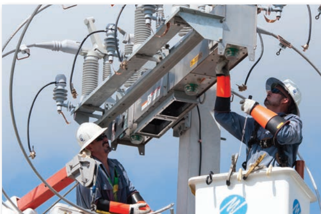
An IntelliRupter fault interrupter being installed.
