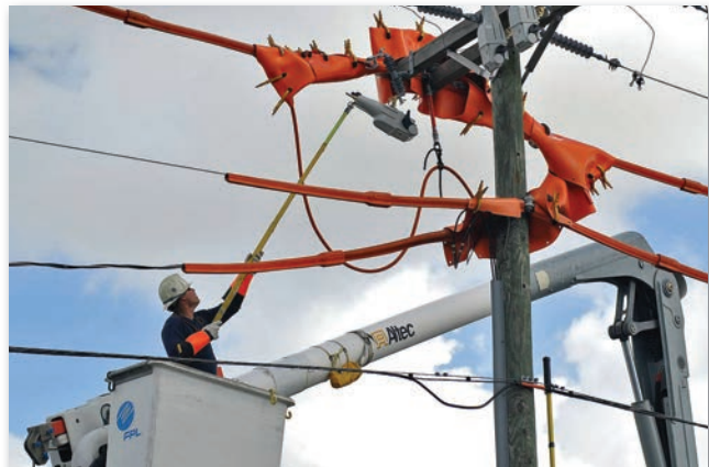
FPL team installs TripSaver II reclosers.
